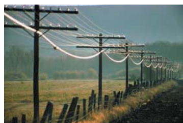
Larry Auippy/Mira.com/Digital Railroad, Inc. A flexible cable suspended between two poles forms a catenary.
